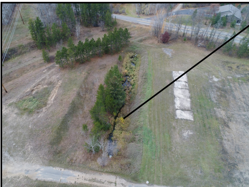
Ditch in natural condition by lake Irving
